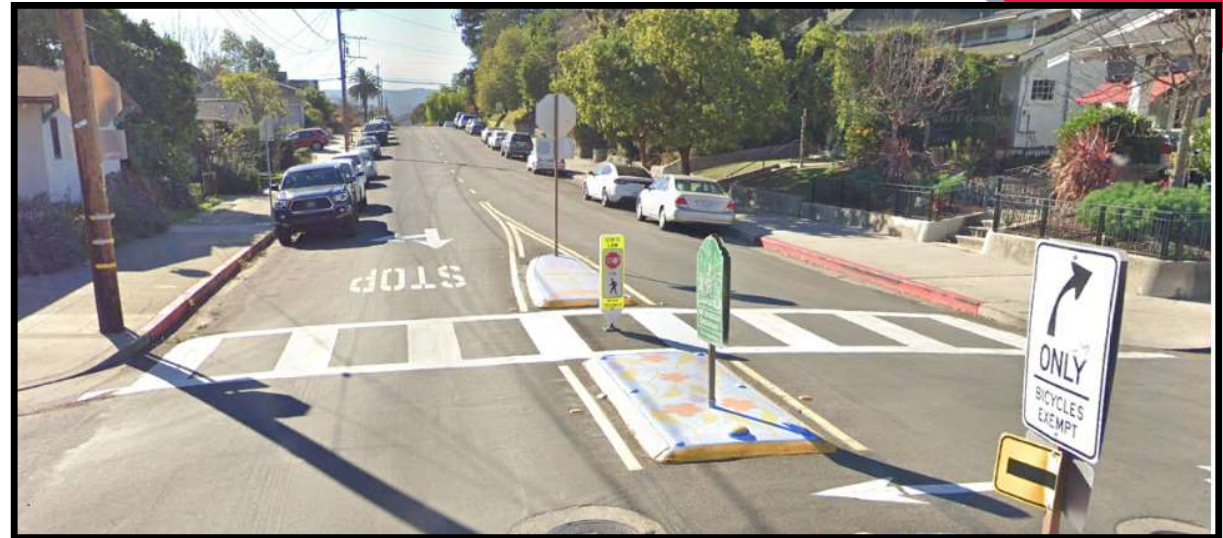
Bike Permeable Median Barrier San Obispo, California
