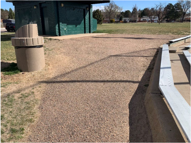
Picture 3: Site of Level Platform, Concrete Wall
